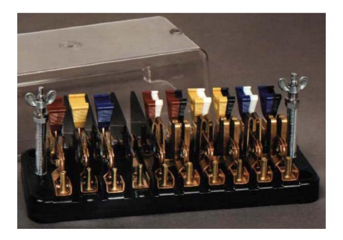
This is an example of a typical 10 pole Safety Test Switch. The 3 knife switches on the left are the voltage phases A, B and C. The 4<sup>th</sup> from the left is the neutral connection for the voltage. The 6 knife switches for the current phases A, B and C are on the right.
